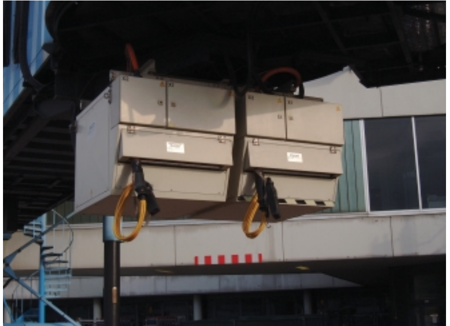
Dual cable coils mounted under a passenger bridge at Fraport, Germany.
